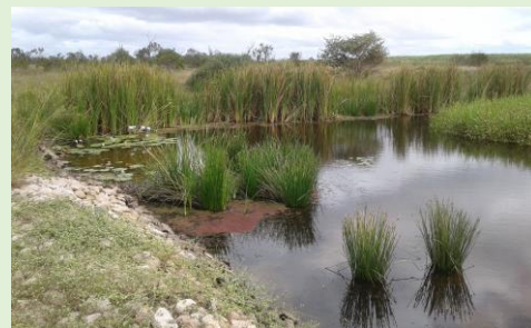
The outlet at the Constructed Wetland Treatment system.
